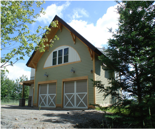
View of the side elevation of the garage with guest cottage above.
