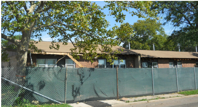
View of existing Parkside Senior construction site.
