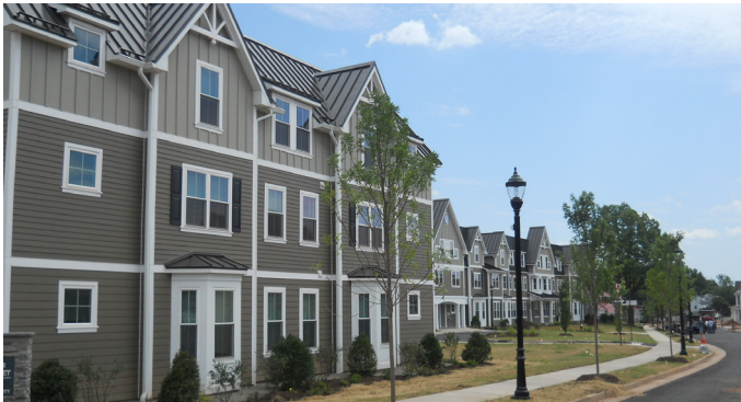
Overall view of the front of the Parkside Senior units.
