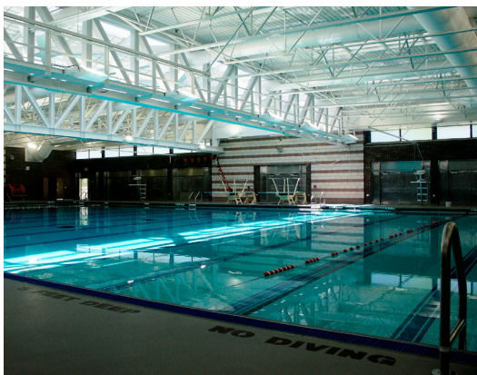
View of the completed Hommock's Pool & Natatorium.
