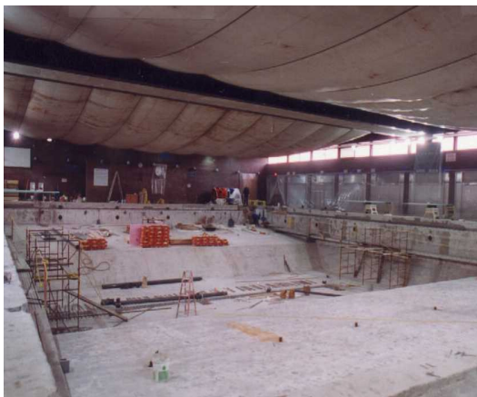
View of the natatorium & swimming pool renovation during construction.
