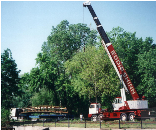
The new bridge being delivered.
