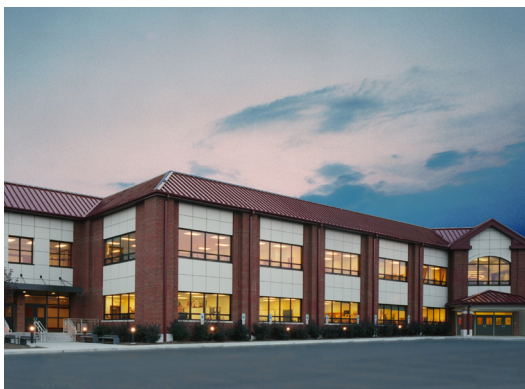
A view of the new addition.
