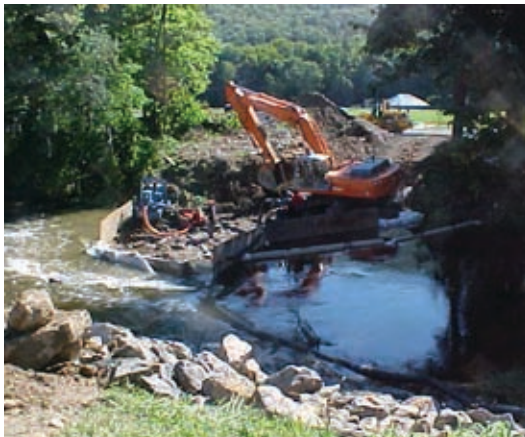
Sewer main replacement through stream bed and flood control levee.
