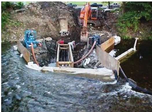
A view of the construction process.
