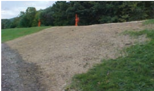
Repaired flood control levee following replacement of sewer main.
